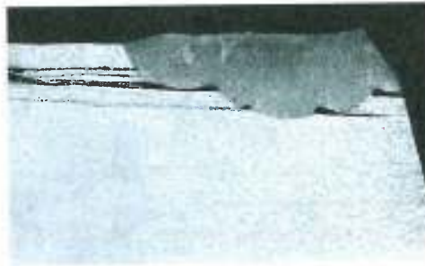
Figure 34-11. Lamellar tearing is caused by welding stresses in the base metal perpendicular to the working direction.
