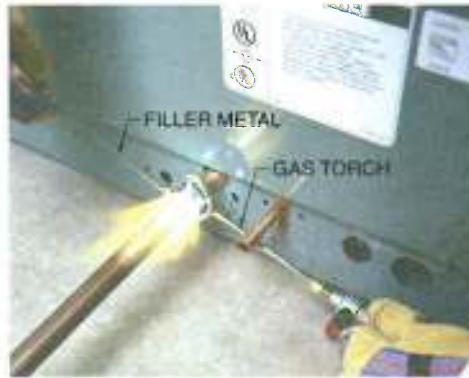
Figure 23-6. A gas torch is commonly used for manual brazing.
