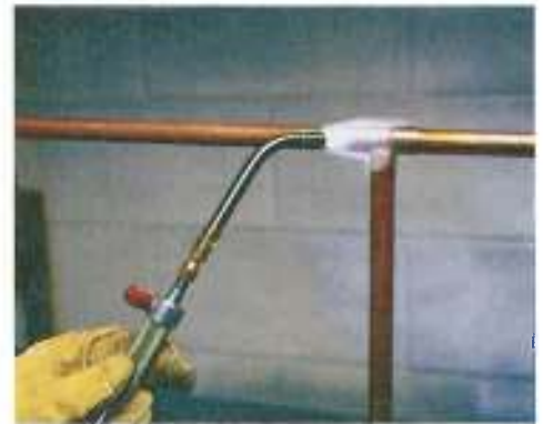
Figure 23-17. A gas torch can be used to solder copper pipe.
