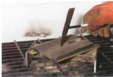
① STRIKE WELD AREA WITH CHIPPING HAMMER
