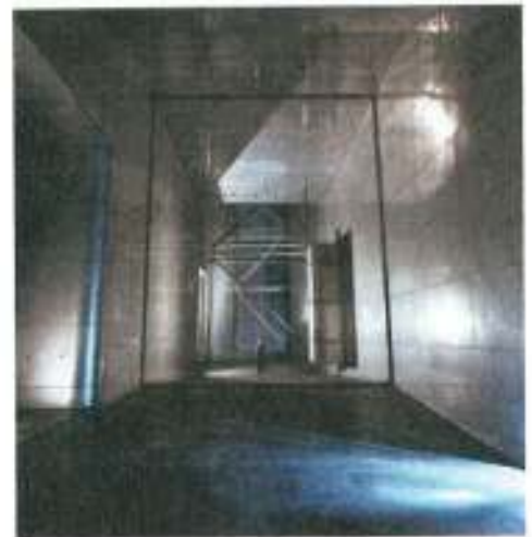
Figure 26-9. Corrosion-resistant sheets are overlapped, with a fillet weld made between new and previously installed sheets, to repair a corroded surface.
